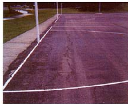
Cracked Asphalt/Hardcourt
